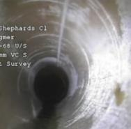
was identified, the pipe could then be cleared of the tree roots and re-lined, so that the drainage system could function again.
