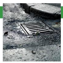
Although we carry out regular drainage cleansing operations, when there are significant amounts of rainfall in a short time, the size of the drainage pipes do not always have sufficient capacity to take all of the water away immediately. Where this happens on a regular basis, we will look at improving the local drainage system by installing wider drainage pipes.
