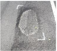
They will next seal the edges and bottom and fill the hole with hot tarmac, spread it and tamp down with a vibrating 'whacker'.
