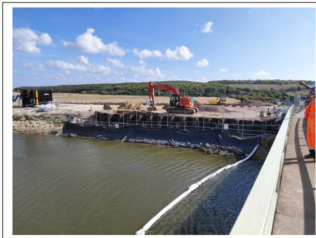
Sheet piling completed on both sides of the river
