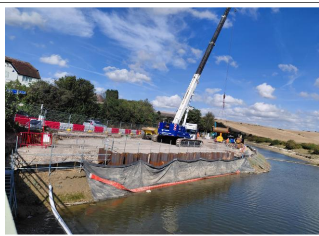
Sheet piling completed on both sides of the river
