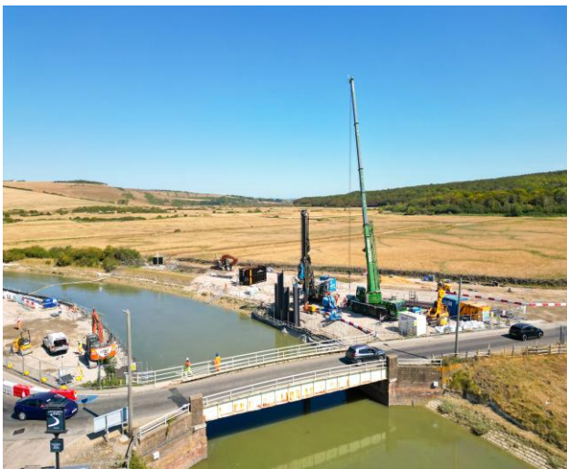
Aerial photo of sheet piling on the east side
