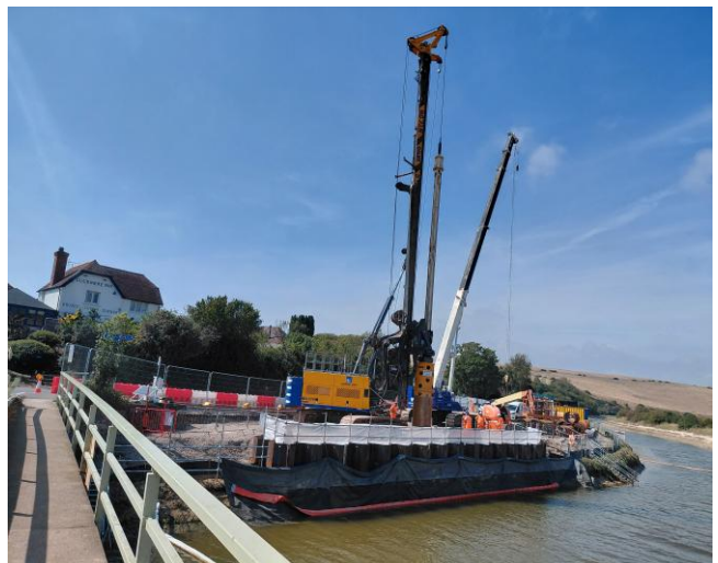
Bored piling rigs are on site to start the test
